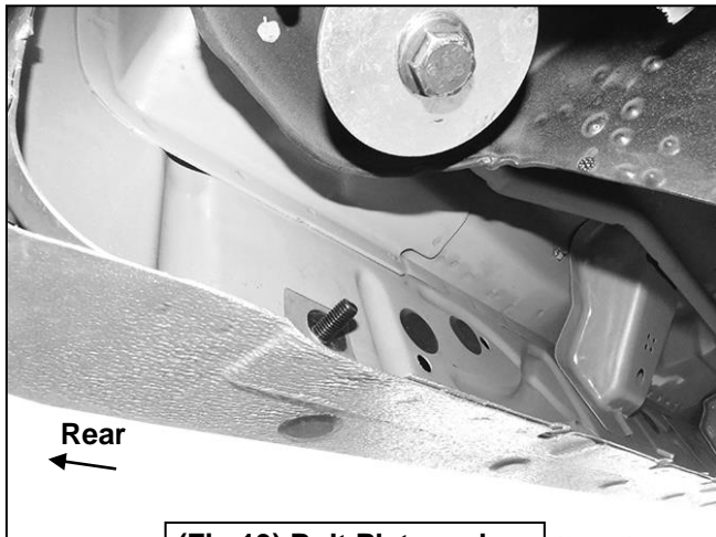
(Fig 13) Bolt Plate and Plastic Retainer installed
