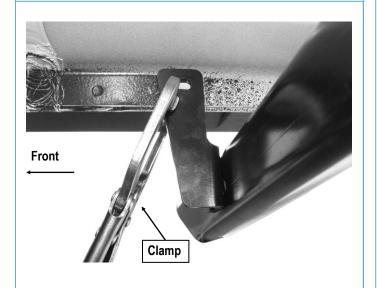
(Fig 6) Use Clamp To Temporarily Hold Front Support Bracket Up To Pinch Weld Until Final Installation
