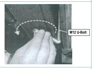
(Fig 2) M12 U-Bolt Installation
