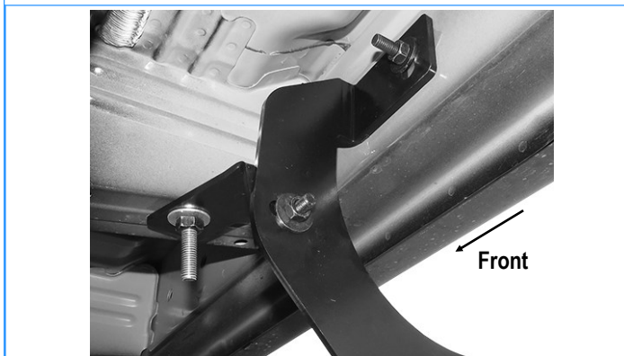
(Fig 9) Passenger Side Center Brackets Installed
