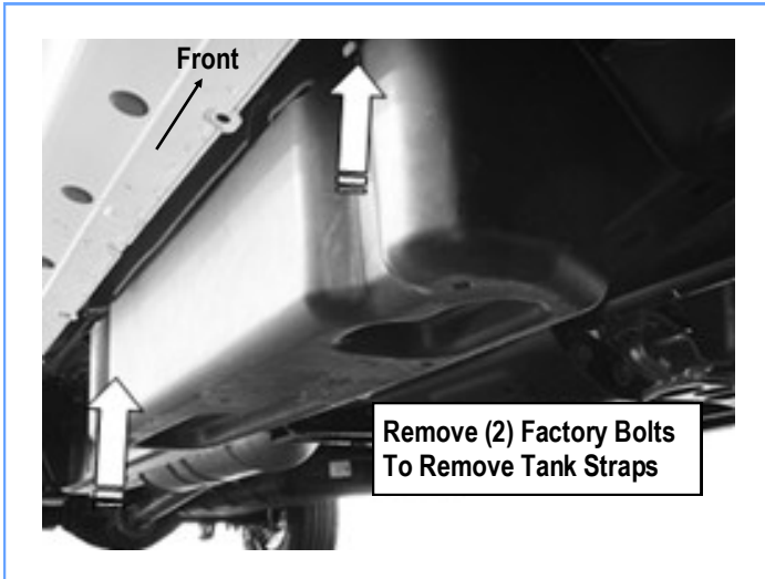
(Fig 11) 07-16 Passenger Side DEF Tank And Cover
