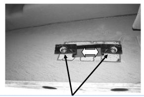
(Fig 2) Slide M8 Clip Nuts Over Holes
