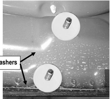
(Fig 2) Thread M8 Plastic Washers Onto (2) Mounting Studs
